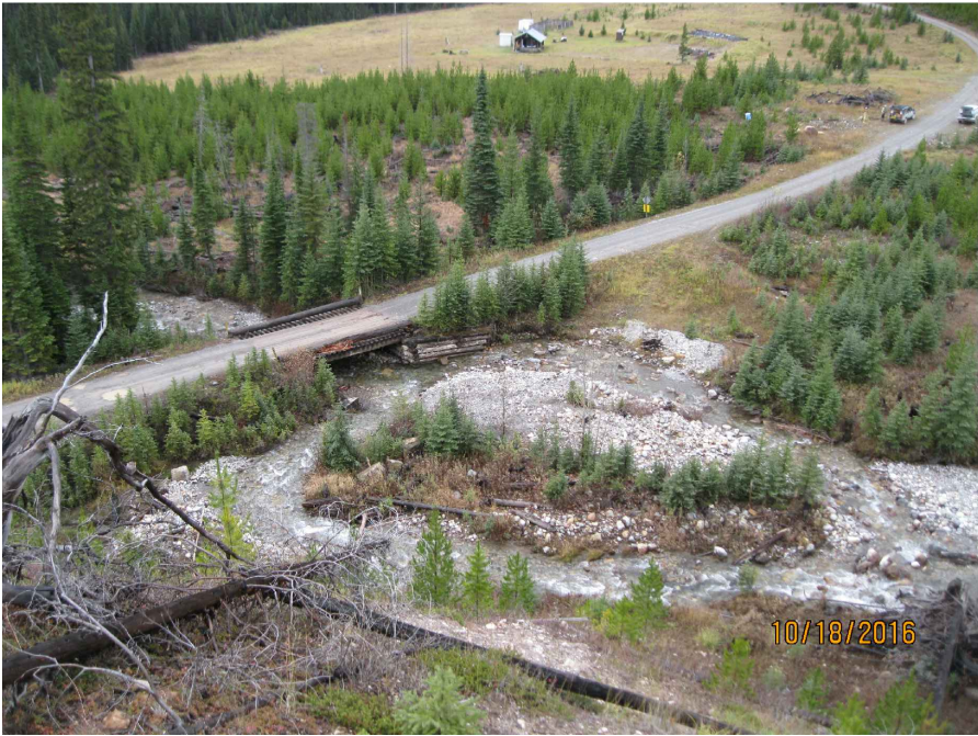
1 10 PHOTO 1 - SITE OVERVIEW SCALE: NTS
