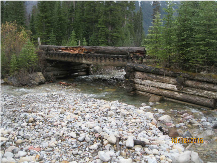
4 10 PHOTO 4 - EXISTING BRIDGE FROM UPSTREAM SCALE: NTS
