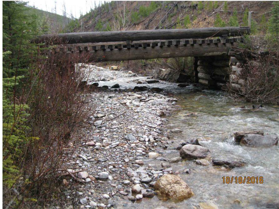
5 10 PHOTO 5 - EXISTING BRIDGE FROM DOWNSTREAM SCALE: NTS
