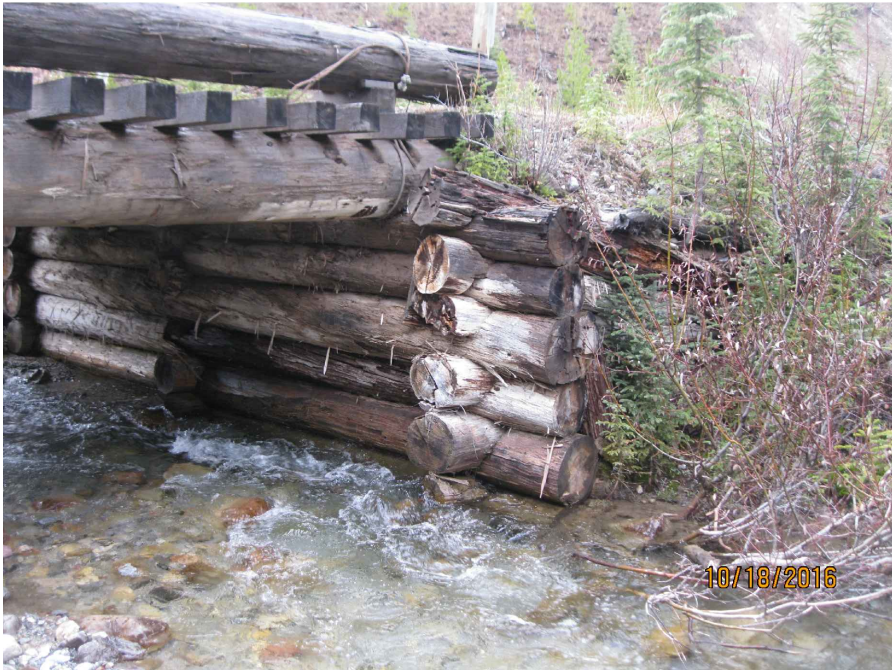
6 10 PHOTO 6 - EXISTING ABUTMENTS SCALE: NTS
